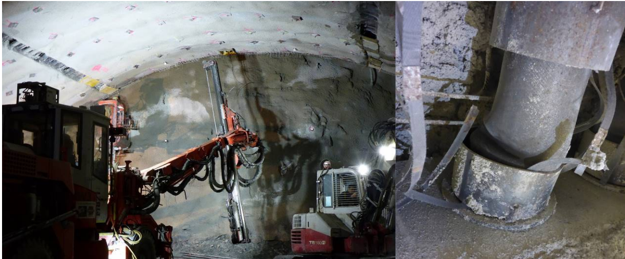
Fig. 5. Lining stress controllers in cavern (source: PGST)
