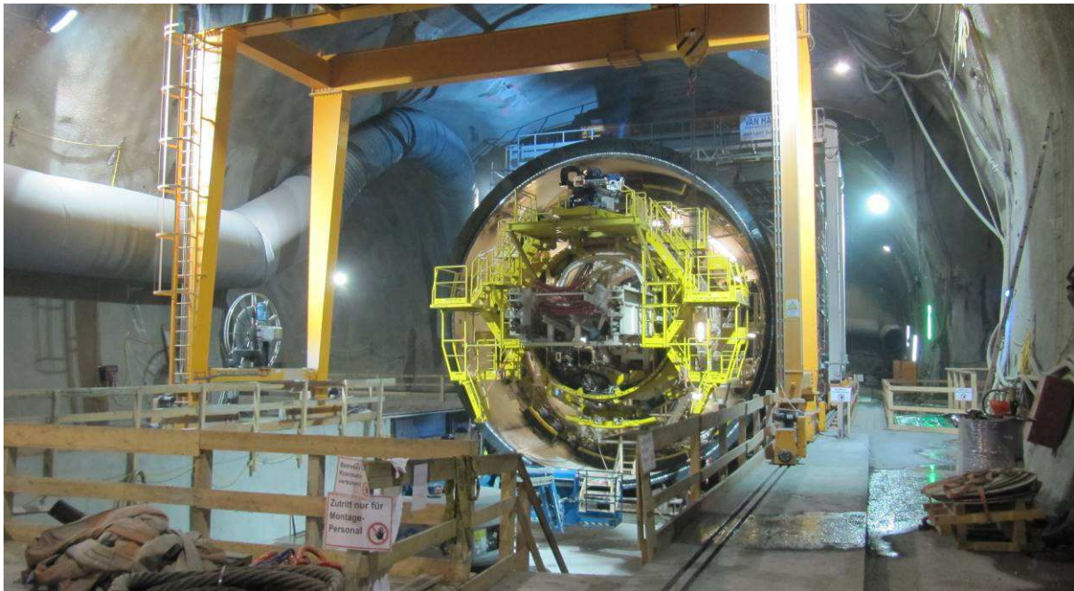
Figure 5: TBM Installation (source: PGST)
