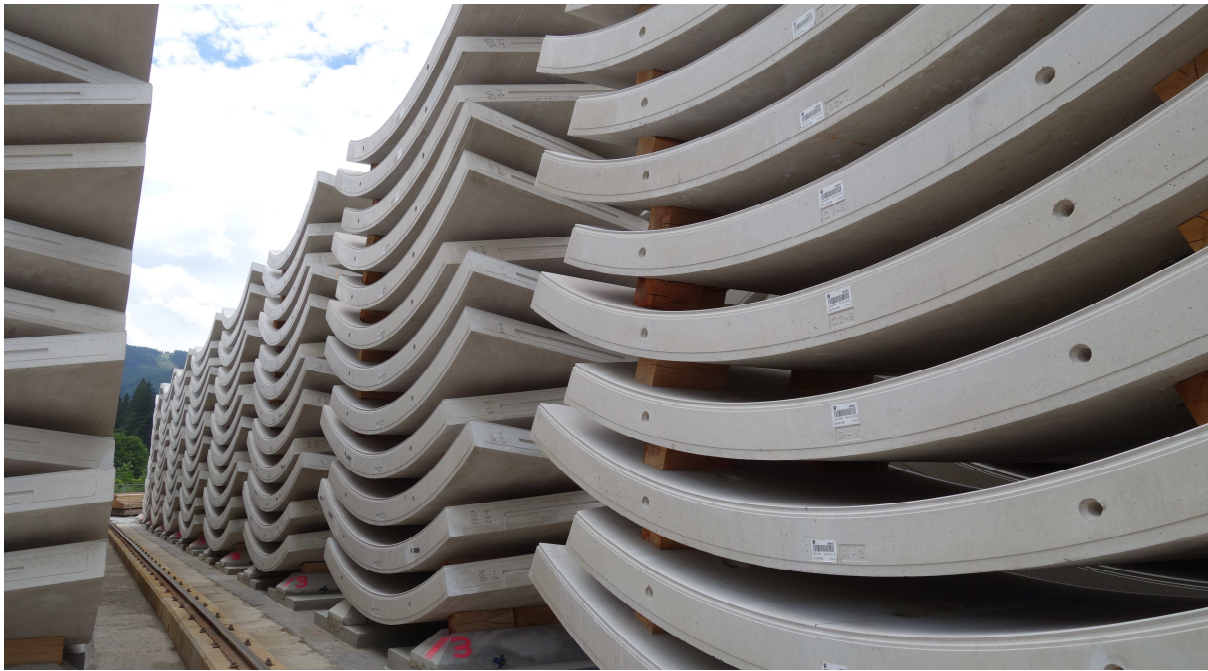
Figure 6: Segmental lining (source: PGST)
