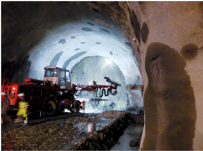
Fig. 3. Twin-track road tunnel with full-face excavation
