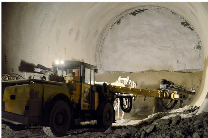
Fig. 5. Single-track railway tunnel with staged full-face excavation
