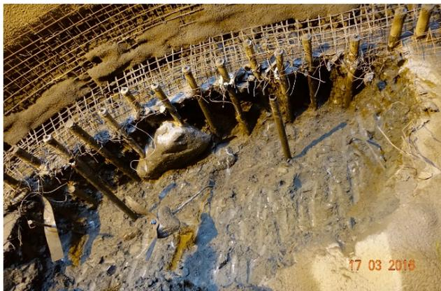
Figure 14: Steel pipes drilled through a boulder
