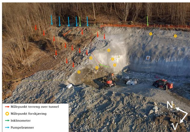
**Figure 13: Location of measuring points, wells and inclinometers**
