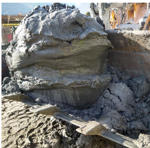
© iC/ Soft, water-saturated lake clay during excavation of bored piles
