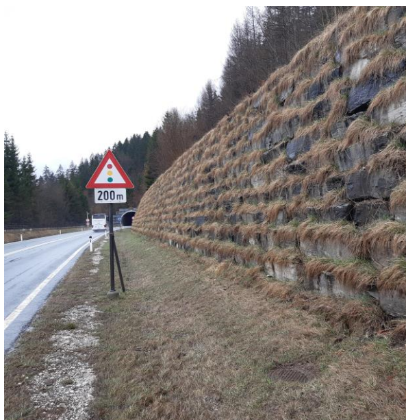
© iC/ Support construction along the B178 before Lärchberg tunnel
