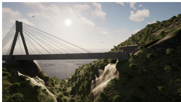
South Portal with main cable-stayed bridge
